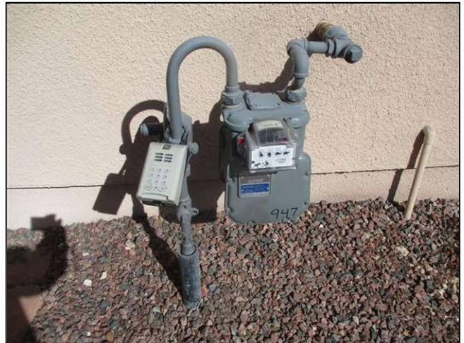
Gas meter / main shut-off
