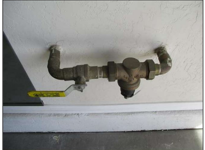
2ndary shut-off / pressure regulator
